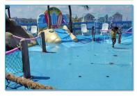
Our Water Flecks® System is comprised of a U.V. resistant Thermo-Plastic Rubber (TPR) mixed with a two-part aliphatic chlorine resistant urethane designed to withstand long-term exposure in chlorinated water.
